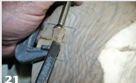
21 The author holds the insert with a C-clamp while chamfering the corners to ease the fit. When dry-fitting the inlay, don't push it in too far, as it will be difficult to remove without damaging it.
