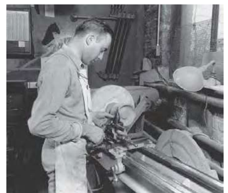
1940s: Prestini worked with a metal lathe. Its gear-driven tool post gave him mechanical control of the forms he created.
